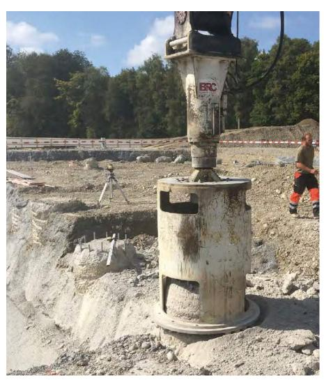
The challenges faced when a perfect pile head is required are manifold! First, the surface tensions must be broken without damage to the surrounding area. This is often done by hand, which is tiring, the working position harmful due to high dust exposure, and there is a high risk of injury to the worker.
